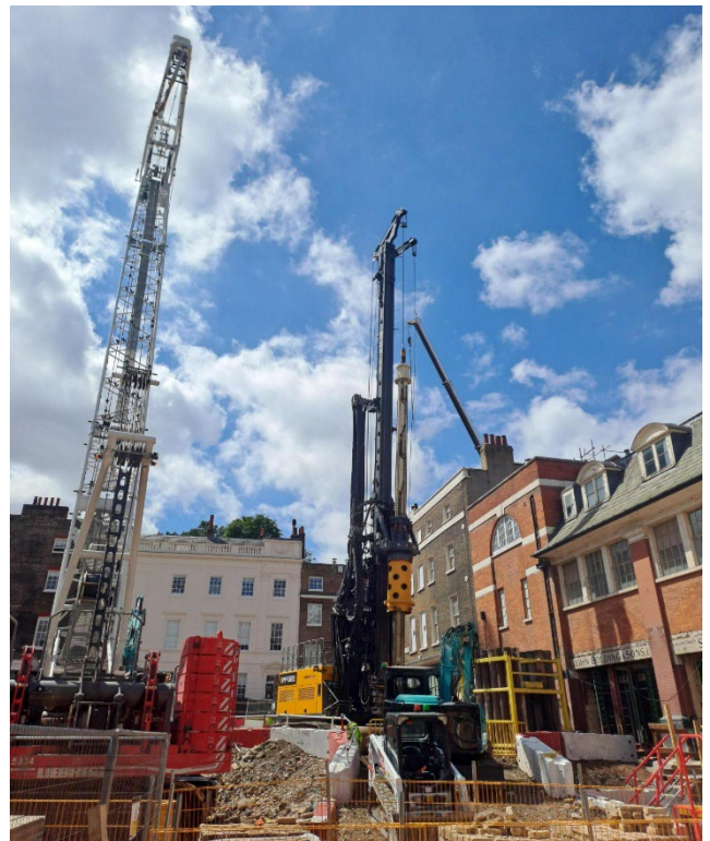
Our Piling Rig and Crawler Crane on site.
