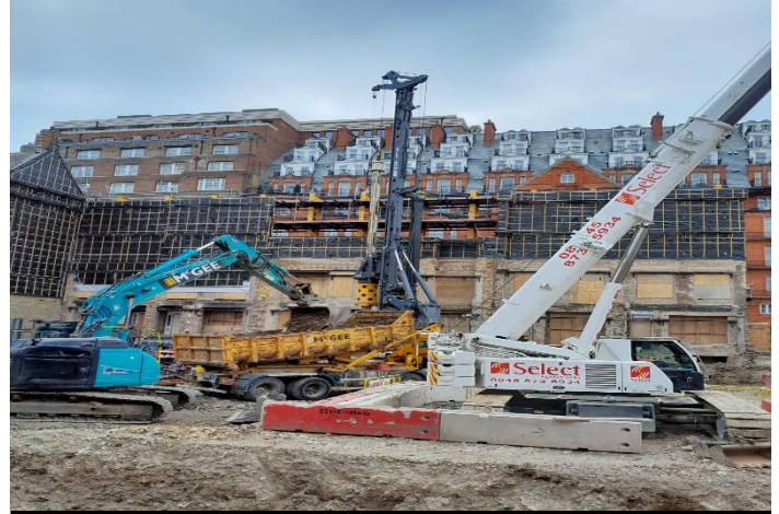
An updated view of the ongoing works on site.
