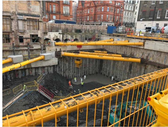
Initial concrete blinding at B2 level
