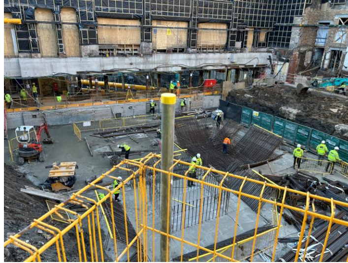
Formation of the lift pits in central slab
