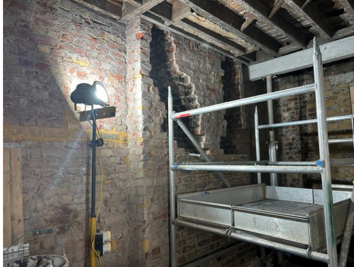
Bricking up of old chimney flues in the RHP
