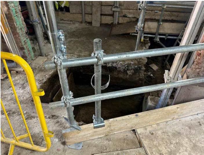
Digging of final underpins
