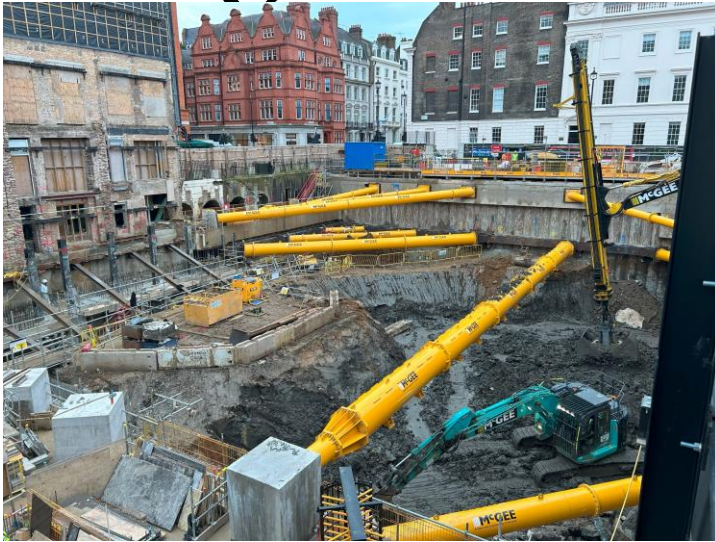
Bulk Excavation down to B2 level
