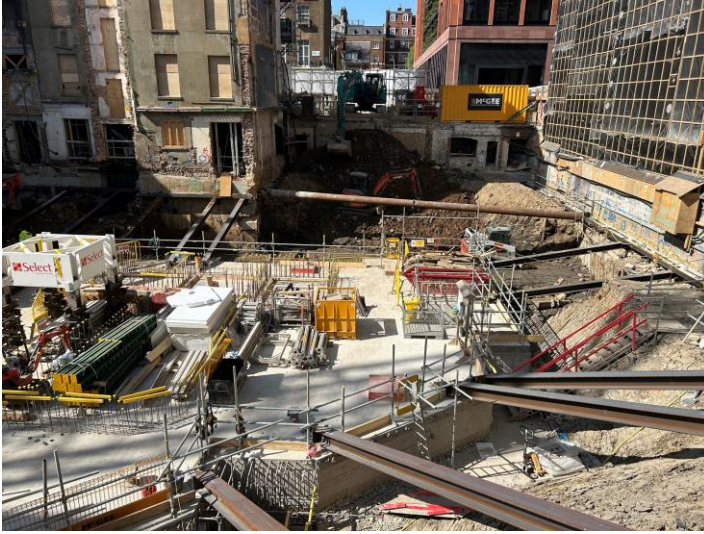
North Block perimeter raking beams
