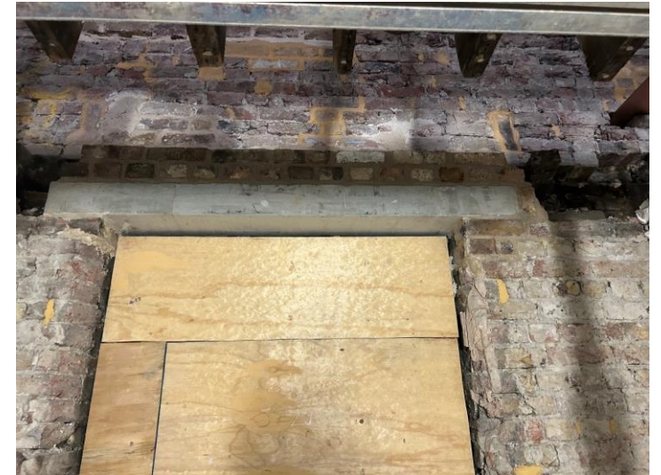
Installation of concrete lintels
