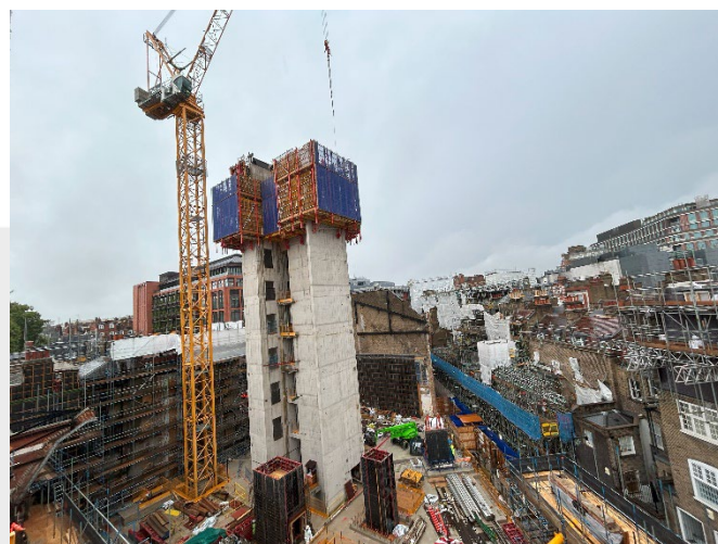
North Block Core progress
