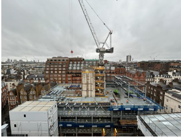
South Structure Progress
