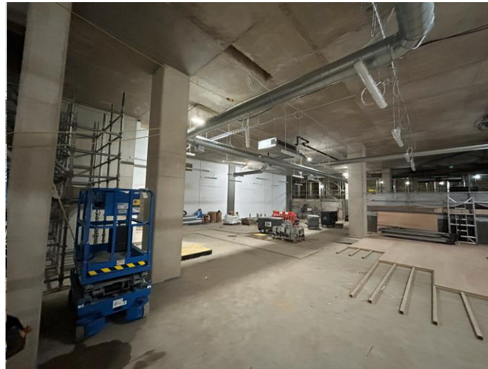
Basement Service Install
