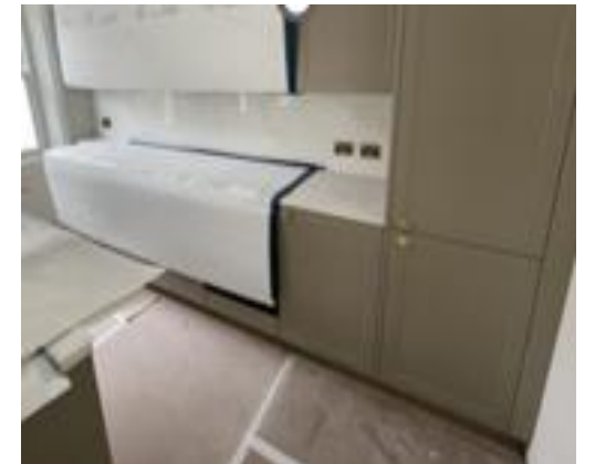
Newly installed kitchen in 16
