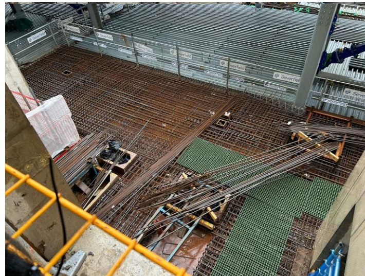
Lobby Slabs Level 1&2 Poured – Level 3 in Progress
