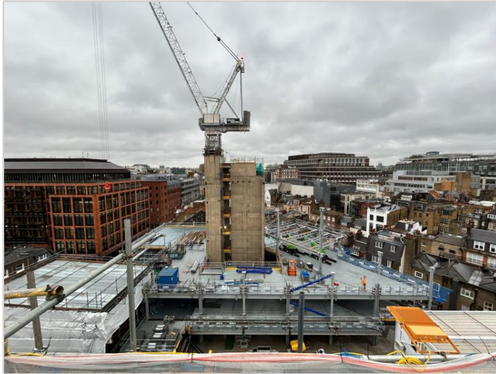
North Structure Progress
