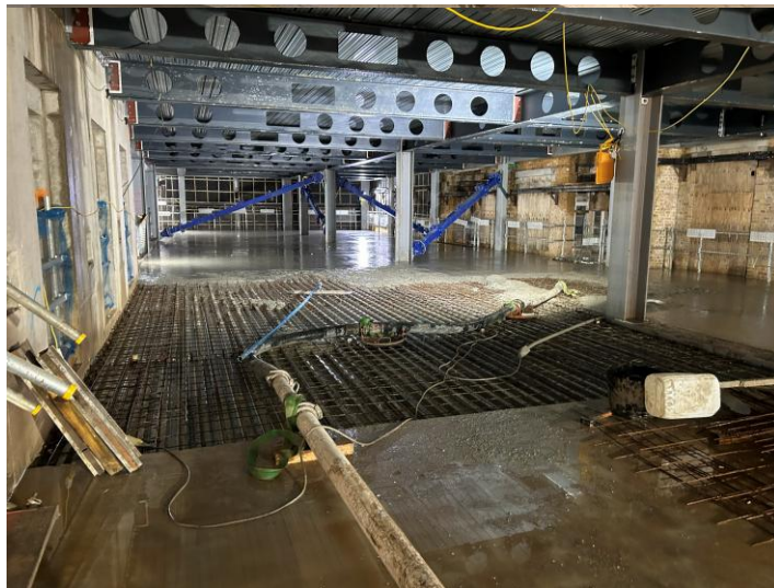
Above Ground Concrete Poured – Level 1
