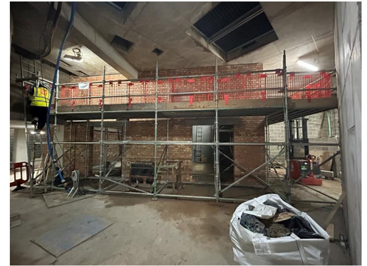
UKPN Room Built
