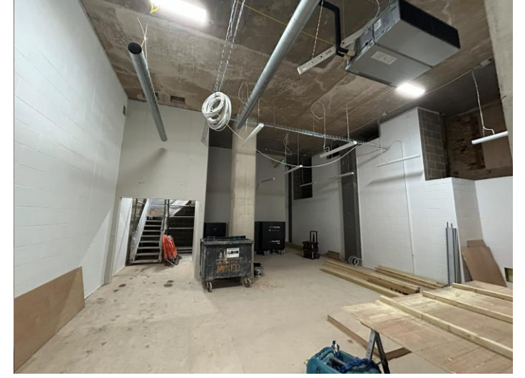
Basement Welfare Fit-Out
